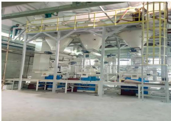
6tph Straw Pellet Line in Bulgaria
