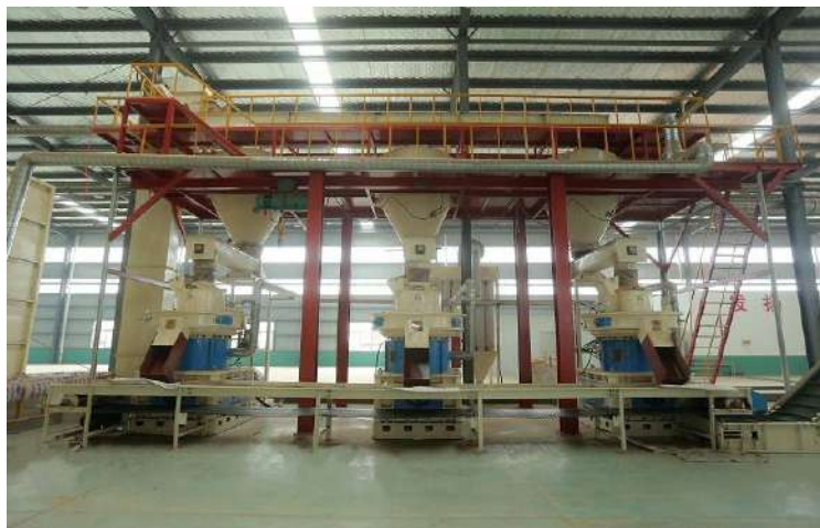
20tph Wood Pellet Line in China
